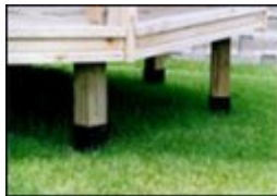
Typical installation of super spikes.
