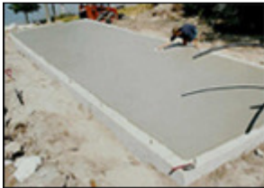
An example of a smooth concrete pad
