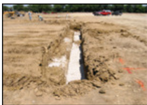
Dig a trench to start building your concrete pad.
